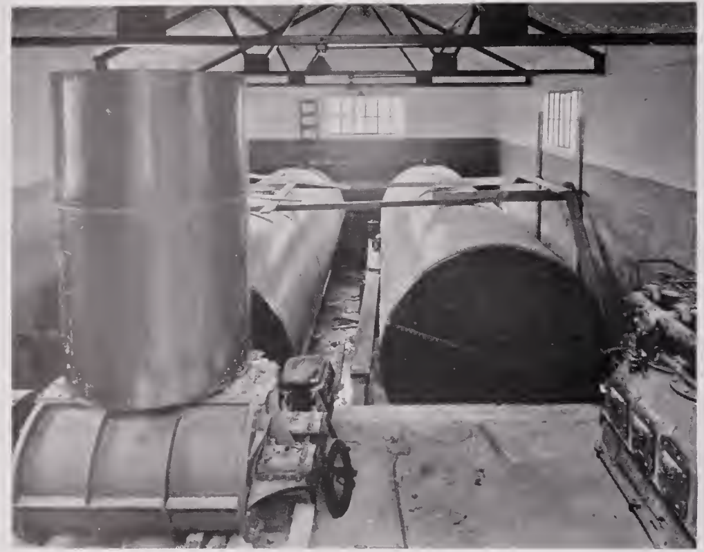
INTERIOR OIL STORAGE BUILDING
